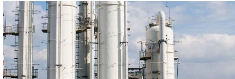
Distillation columns at the JSR chemical plant. (Source: JSR Corporation)
