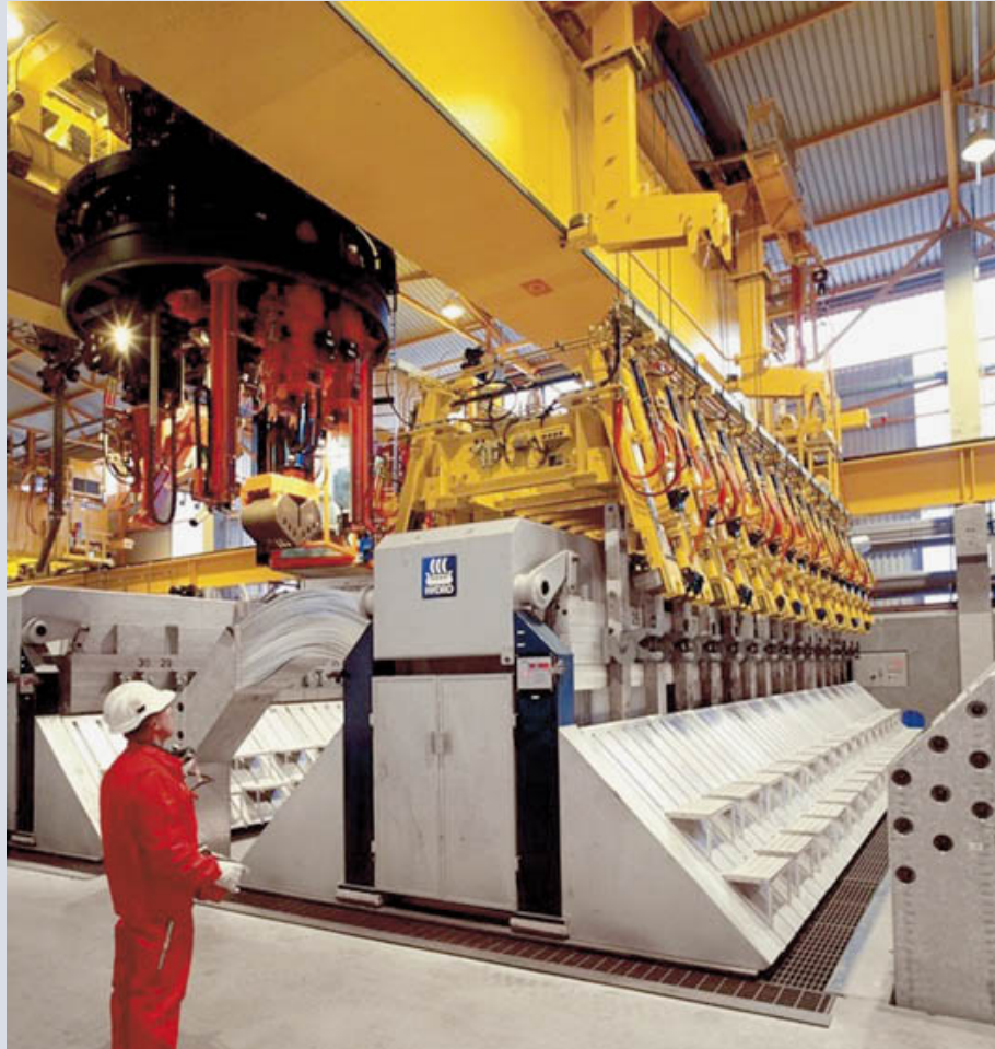
Fig. 2: Crane system for electrodes
