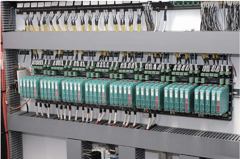
Fig. 2: Fieldbus power supplies with physical layer diagnostics
