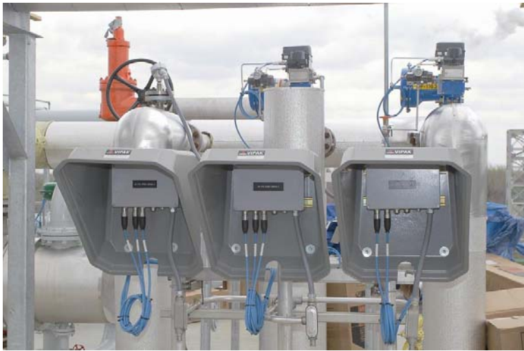
Fig. 3: FieldBarrier with FISCO spur connections
